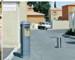
Access control unit
